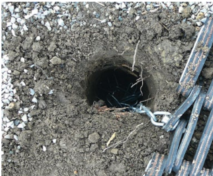
Small hole in ground for anchor chains + point foundation (approx. Ø 5.00 cm)
