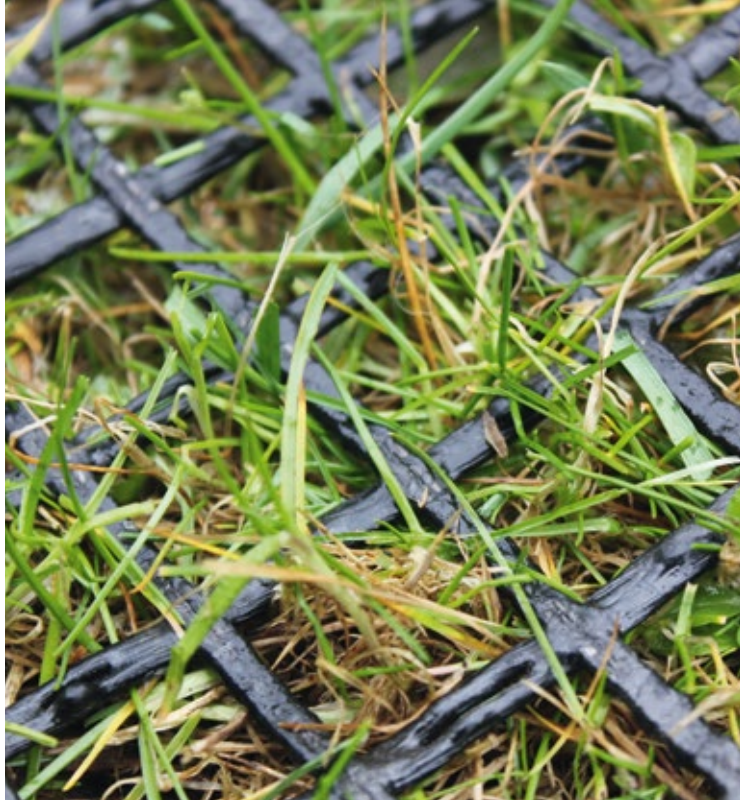
Mats approx. 4-5 weeks after installation
