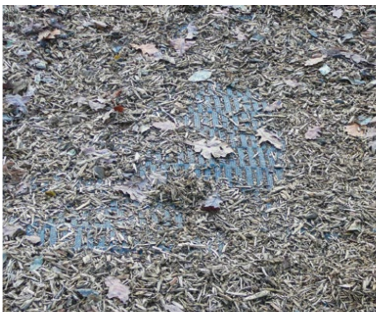
Lawn protection mats after installation (laid open for photo)
