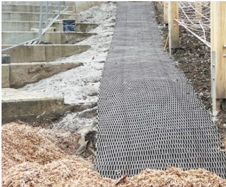
Mats directly after laying
